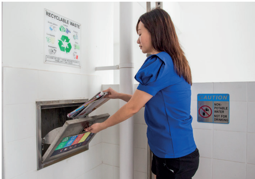
Separate chutes for recyclable waste
