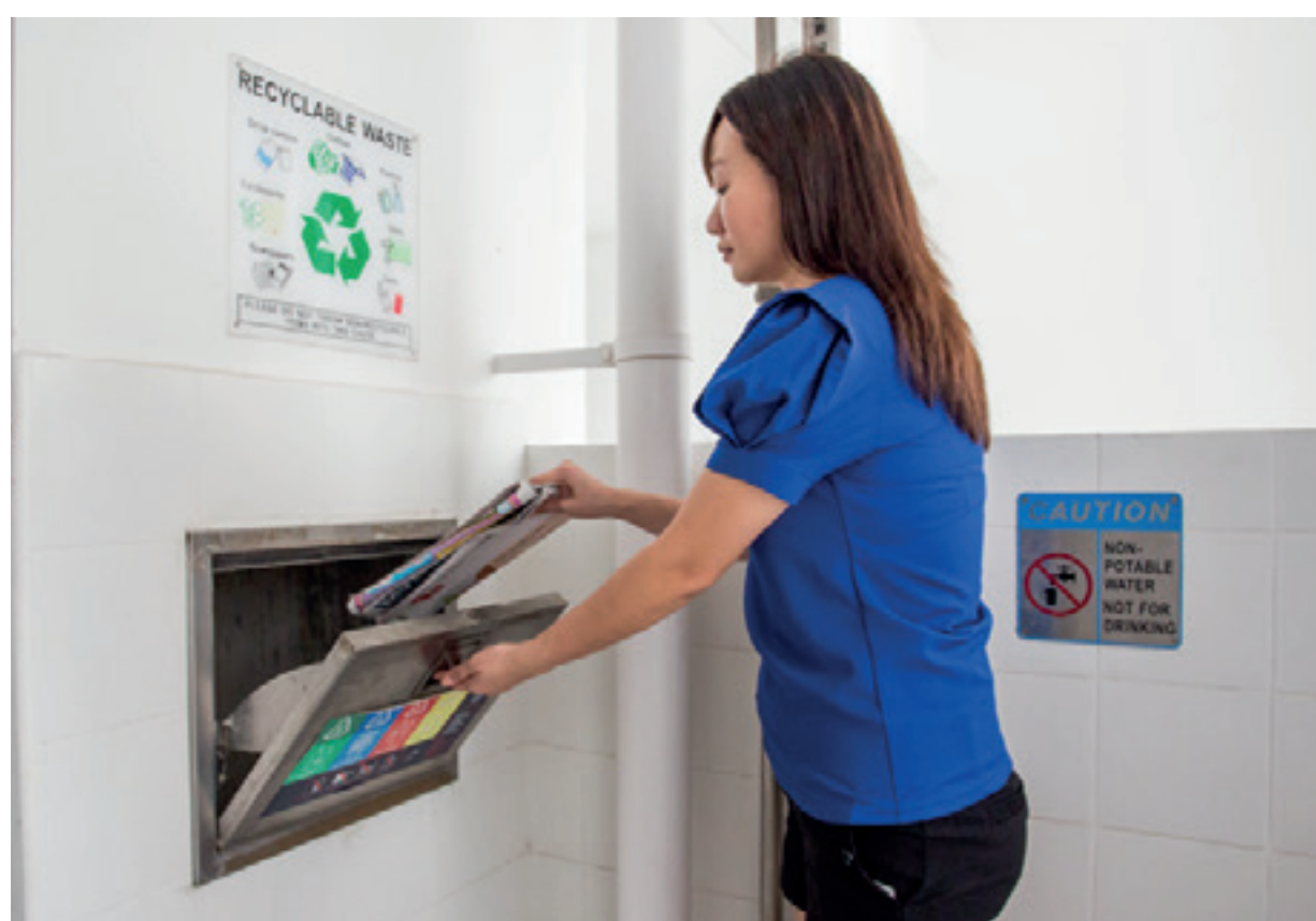
Separate chutes for recyclable waste
