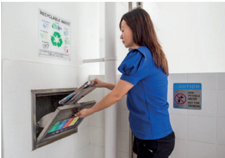
Separate chutes for recyclable waste
