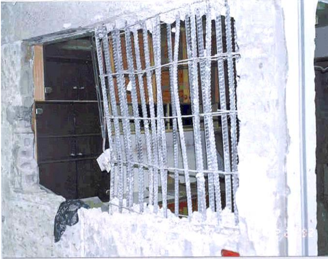
Exposed reinforcement bars
