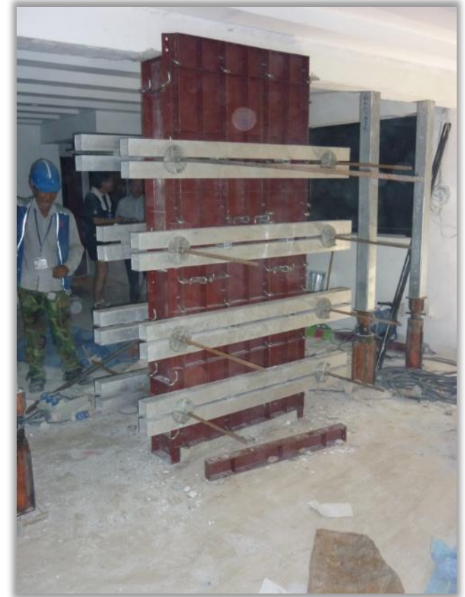
Repair works for hacked structural column
