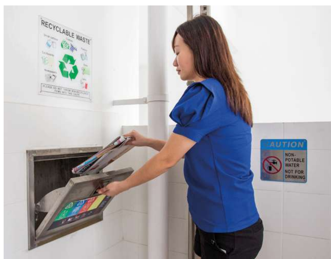
Separate chutes for recyclable waste
