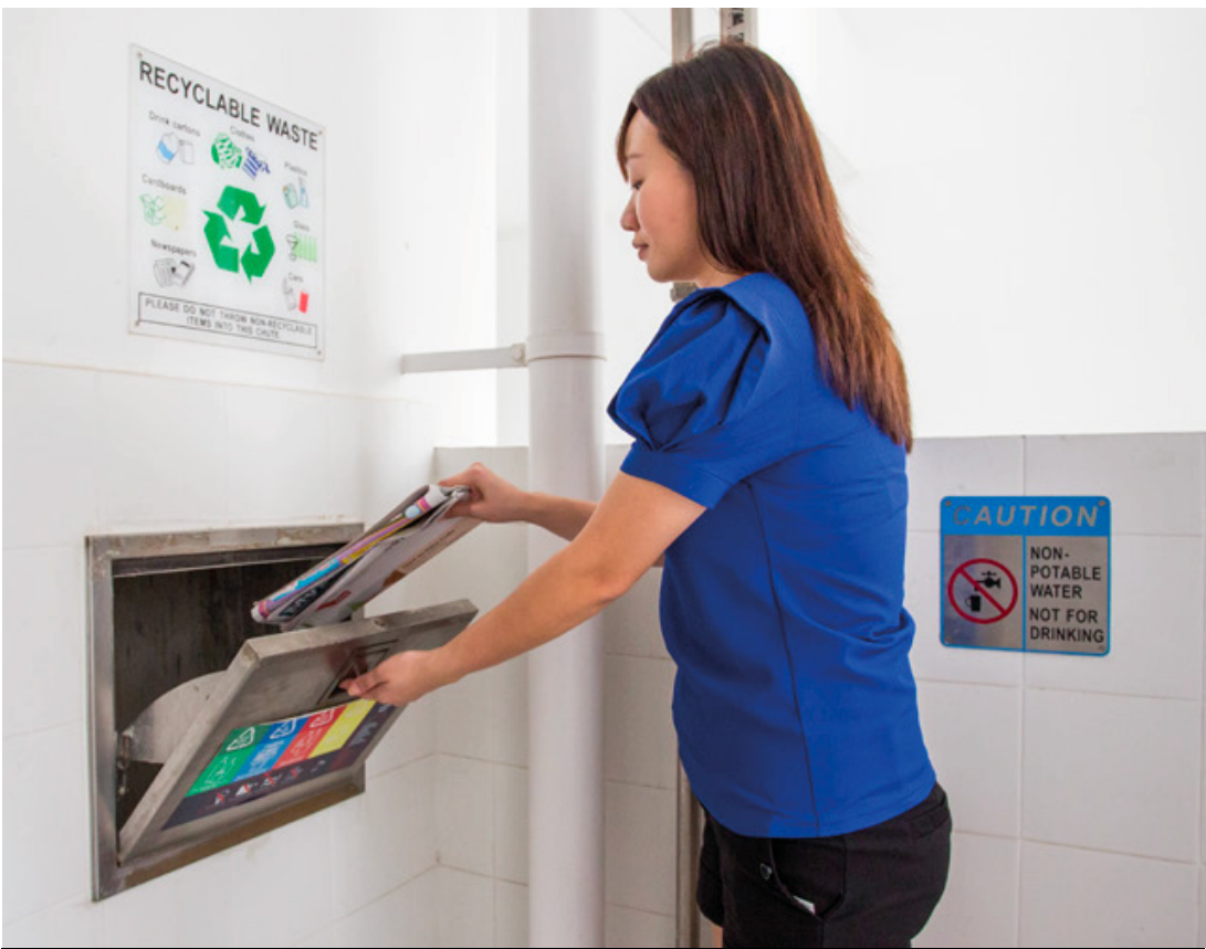
Separate chutes for recyclable waste
