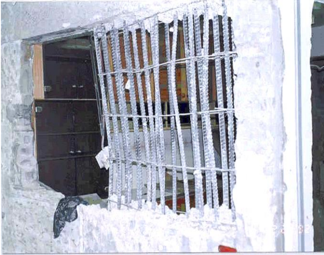
Exposed reinforcement bars
