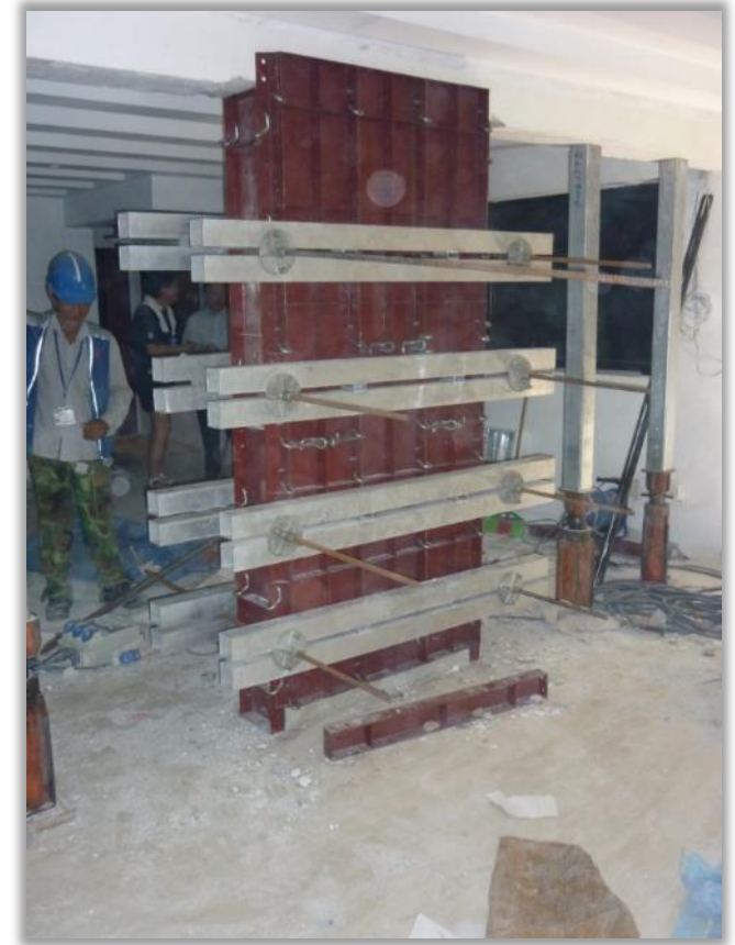
Repair works for hacked structural column
