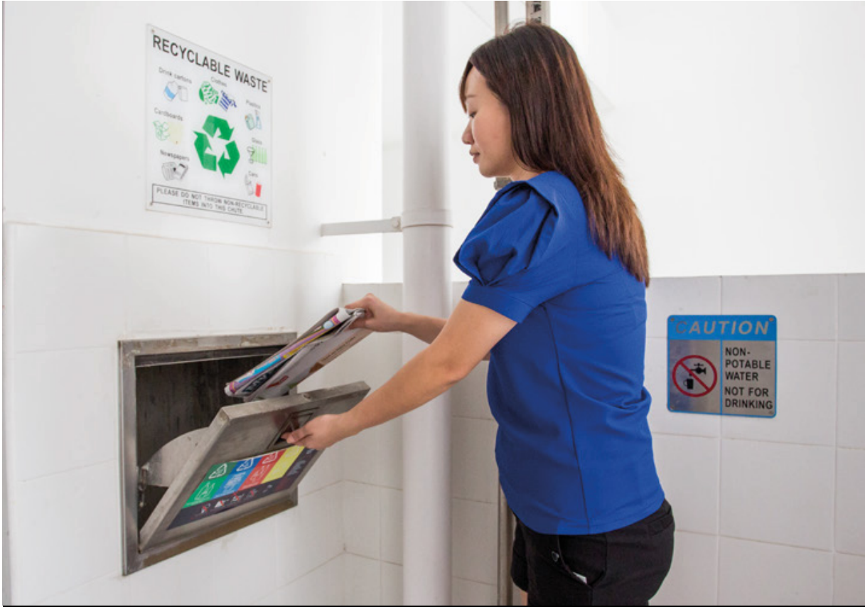
Separate chutes for recyclable waste
