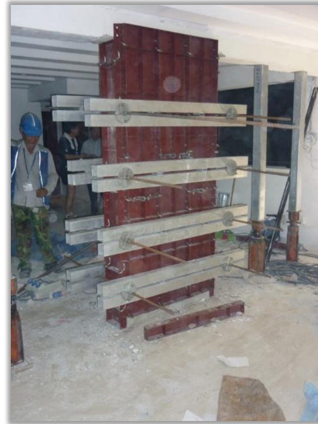
Repair works for hacked structural column
