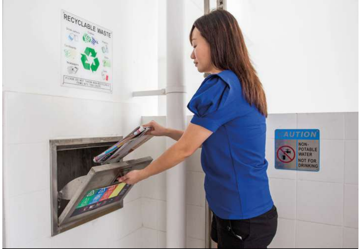
Separate chutes for recyclable waste
