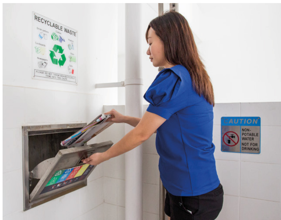
Separate chutes for recyclable waste
