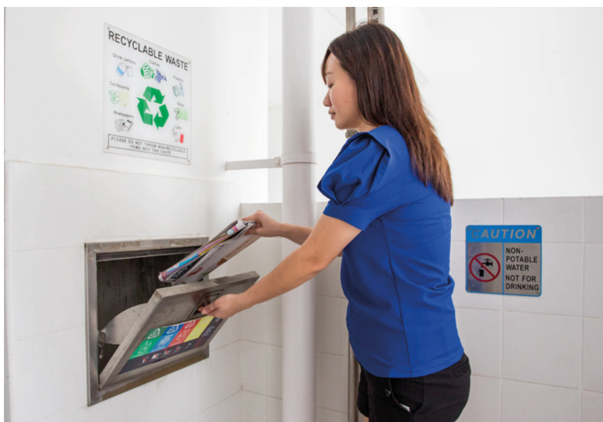
Separate chutes for recyclable waste
