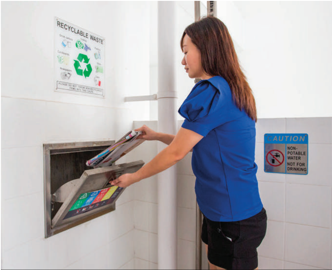
Separate chutes for recyclable waste
