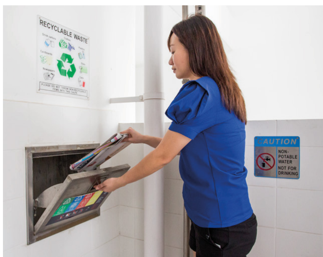
Separate chutes for recyclable waste
