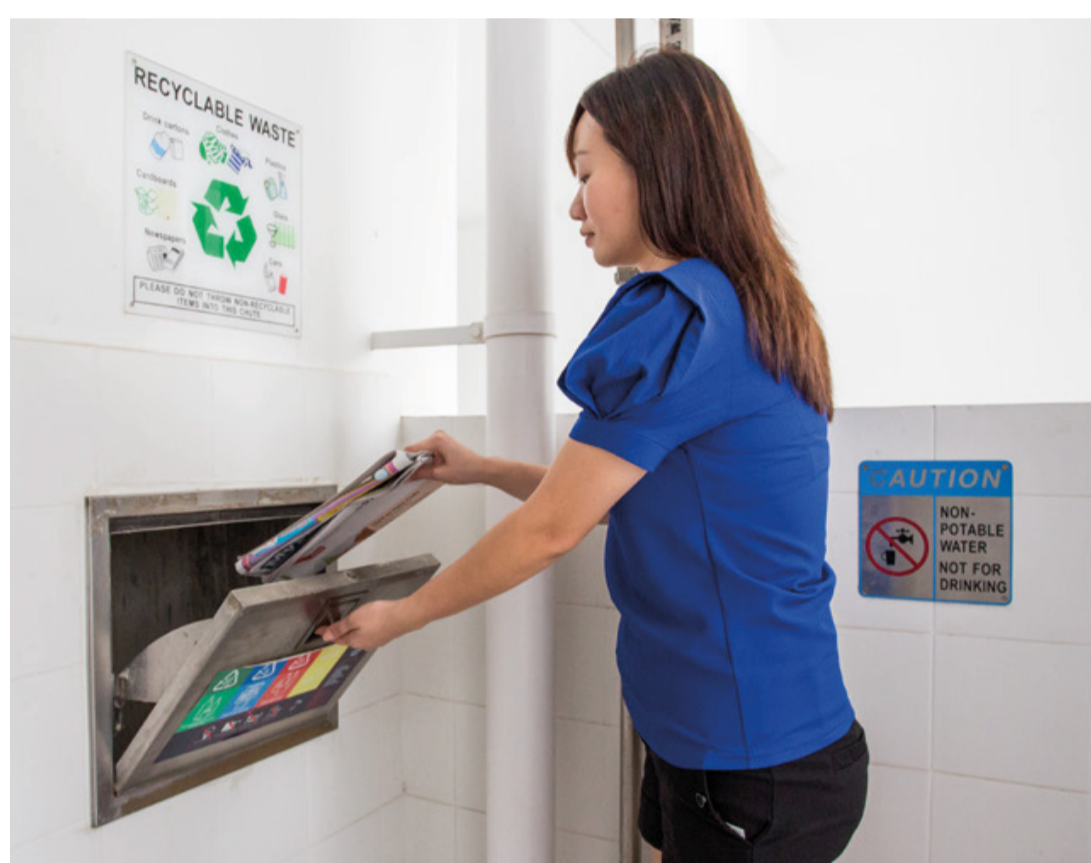
Separate chutes for recyclable waste
