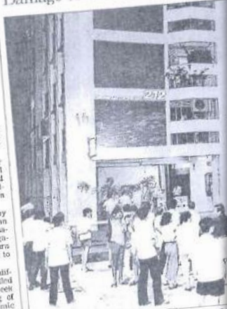
Residents from nearby blocks milling around a column room and flat.
