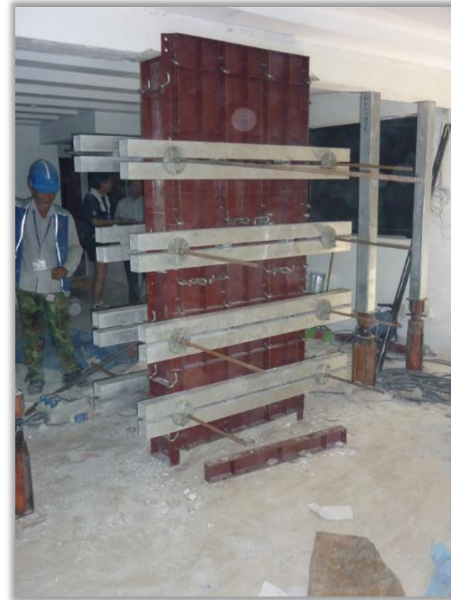
Repair works for hacked structural column
