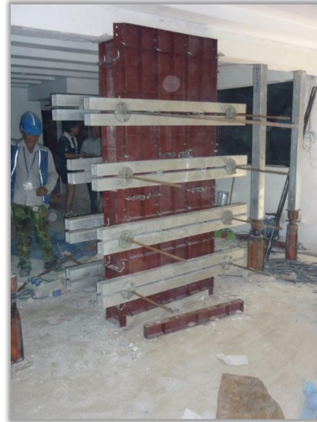
Repair works for hacked structural column
