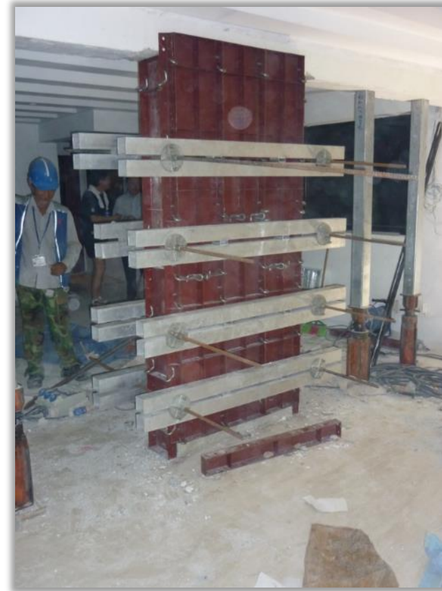
Repair works for hacked structural column
