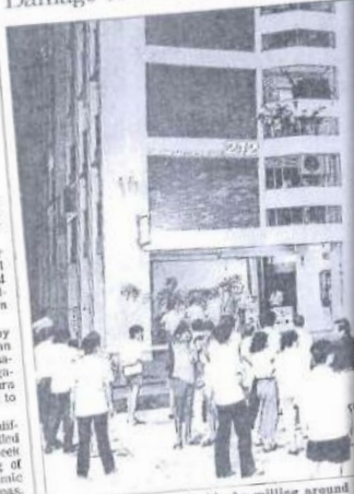
Residents from nearby blocks milling around a column room and flat.
