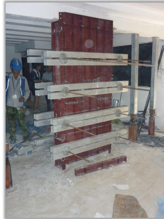
Repair works for hacked structural column
