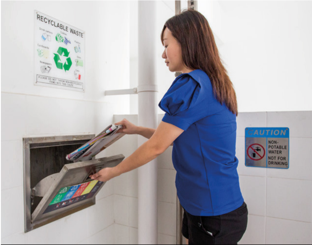
Separate chutes for recyclable waste
