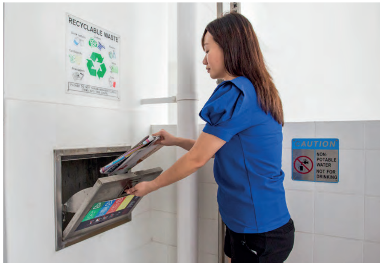
Separate chutes for recyclable waste
