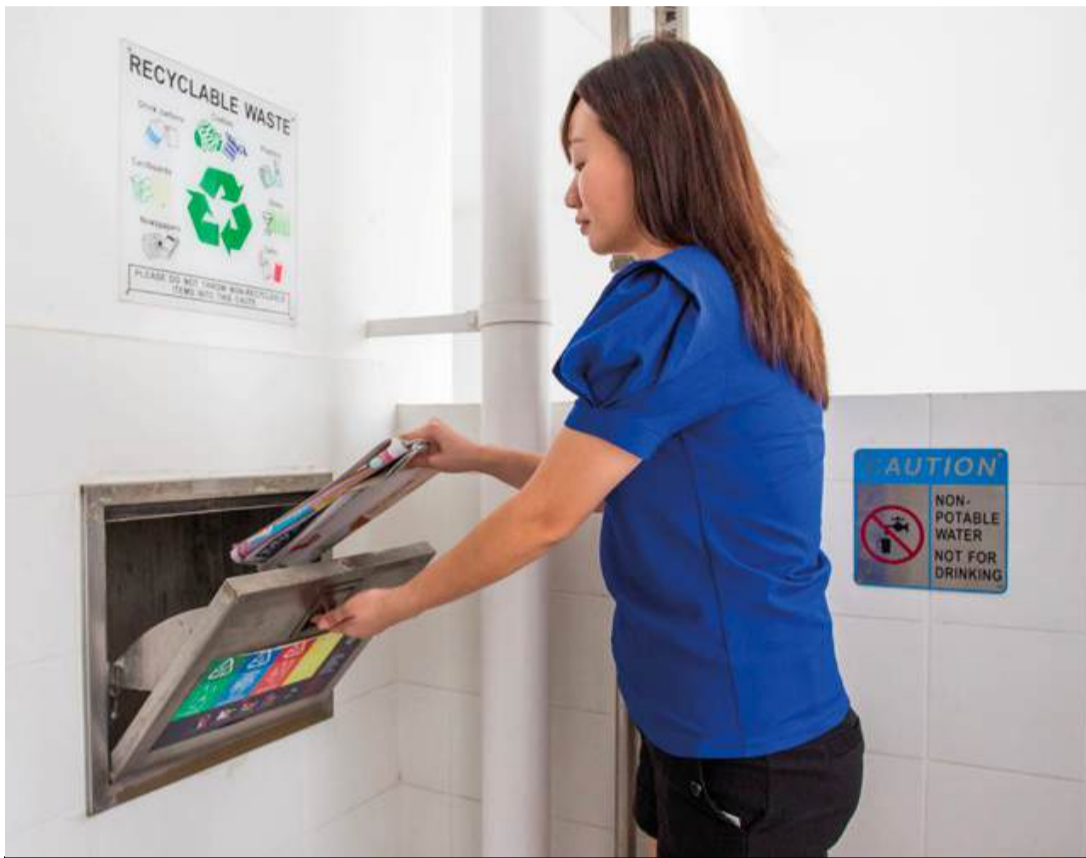
Separate chutes for recyclable waste
