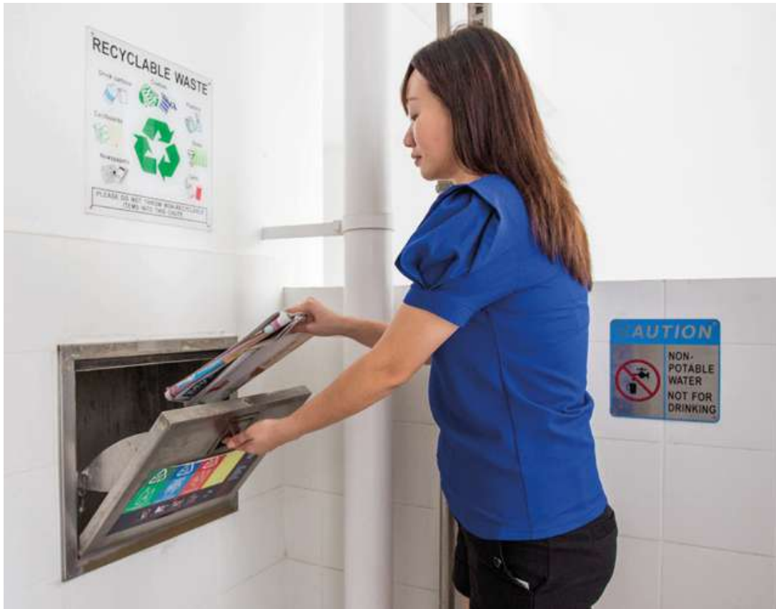
Separate chutes for recyclable waste
