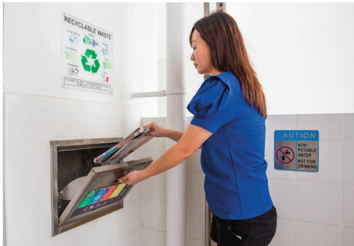
Separate chutes for recyclable waste
