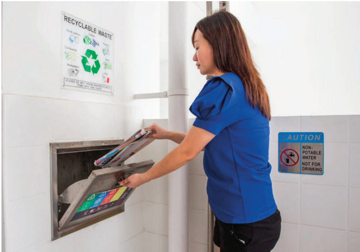
Separate chutes for recyclable waste
