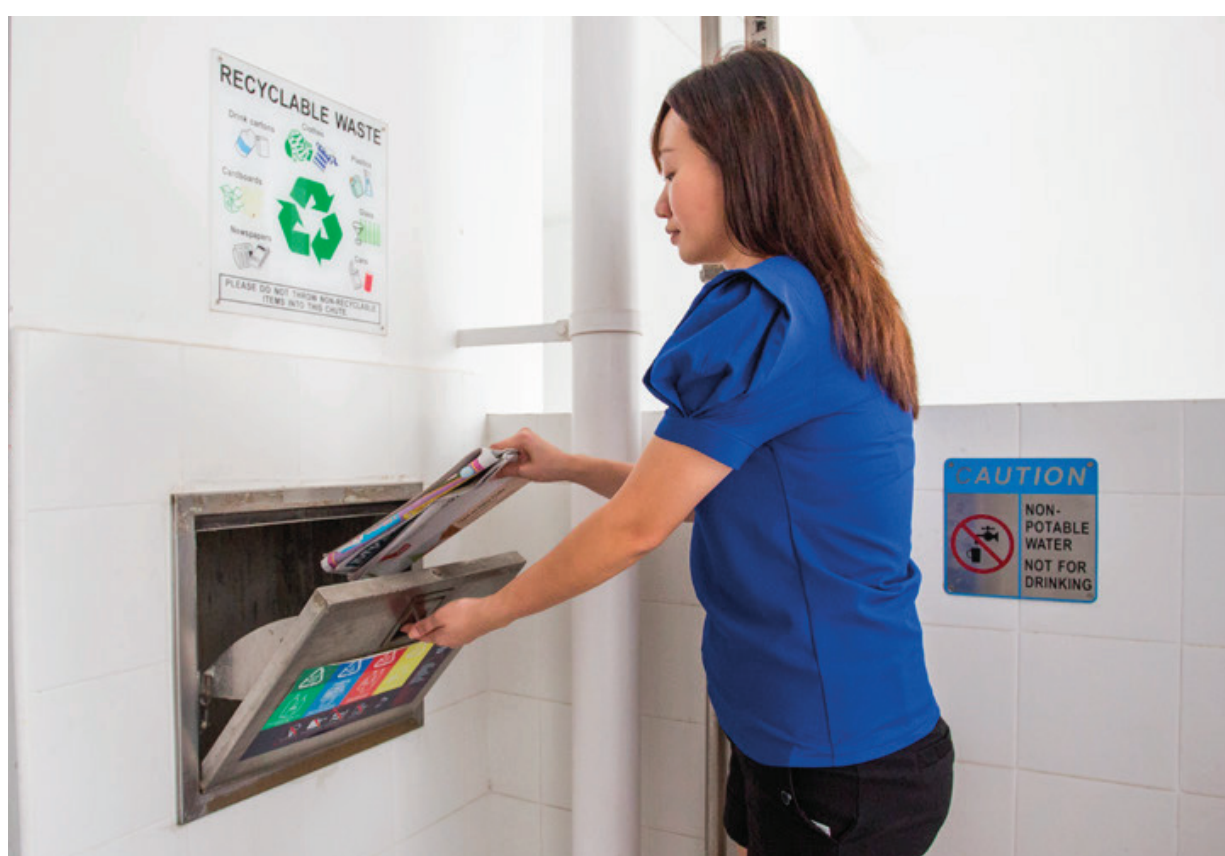
Separate chutes for recyclable waste
