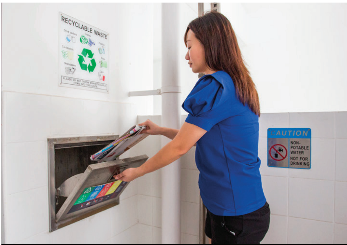
Separate chutes for recyclable waste
